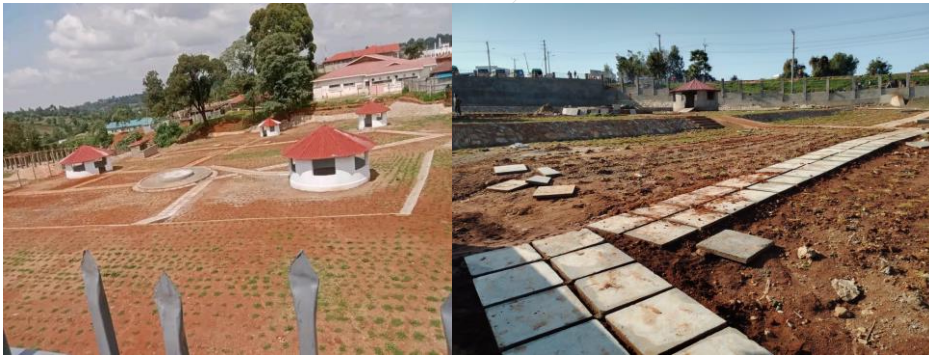
Figure 1: Ongoing construction of Makutano recreational park
