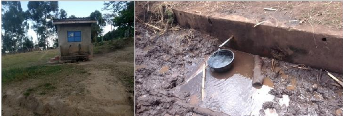
Plate 13: Left_ is unused borehole in Keringet village. Right_ a drying water source in Kaprech.
