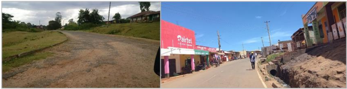
Plate 4: Left_ is the Status of roads in Bendera Town. Right_ is a road in Makutano town lacking other road elements.
