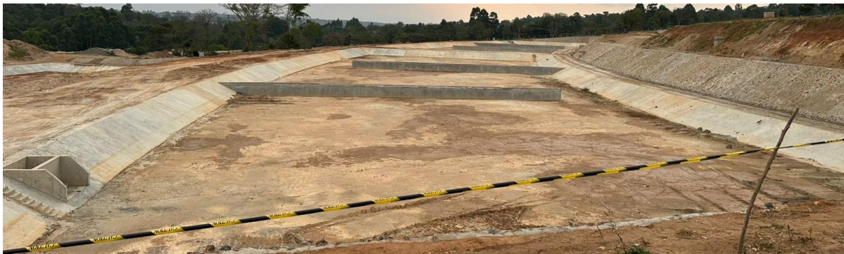
Plate 28: Sewerage project in Lityei
