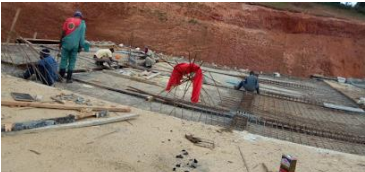
Plate 12: Muruny water supply project (under construction)
