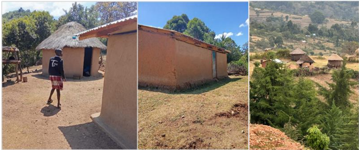
Plate 20: Mud-Wall material in Kapenguria Municipality
