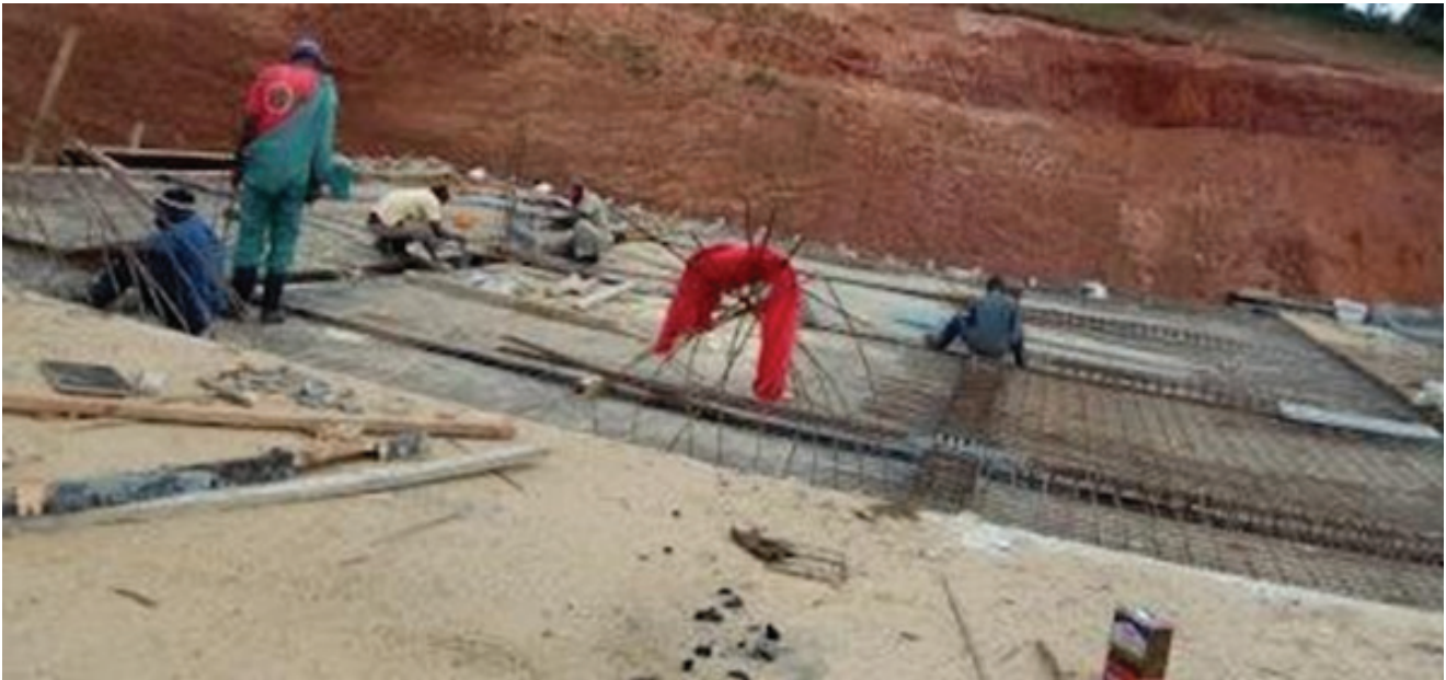
Plate 6: Muruny water supply project (under construction)
