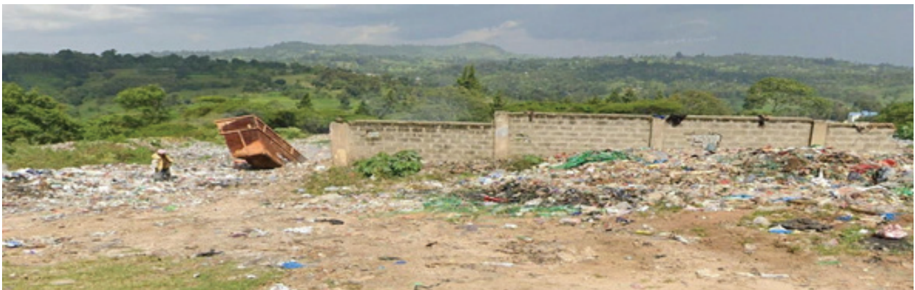
Plate 15: Kapenguria Dumpsite, existing fence. Source: Field Survey, 2023.
