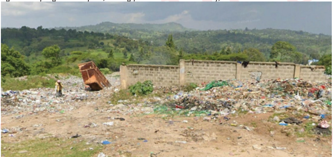
Figure 9: Kapenguria Dumpsite, existing fence. Source: Field Survey, 2023
